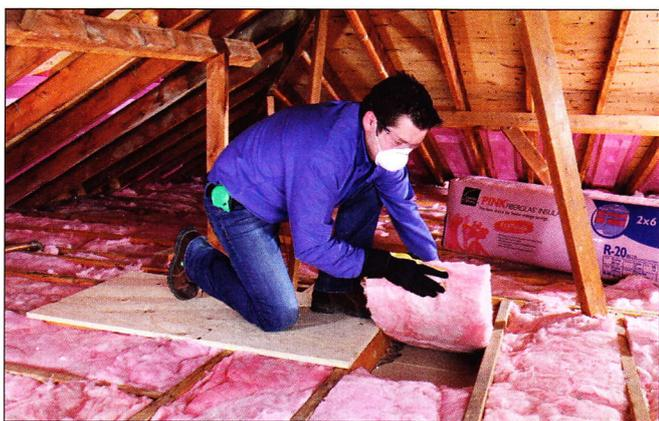
Manufacturers have been keeping a close eye on the move to Energuide 80. In January, Owens Corning Canada launched EcoTouch PINK FIBREGLAS insulation to replace its traditional product. This batt insulation contains over 70 per cent recycled content, making it a sustainable way to match or exceed Energuide 80 standards.
